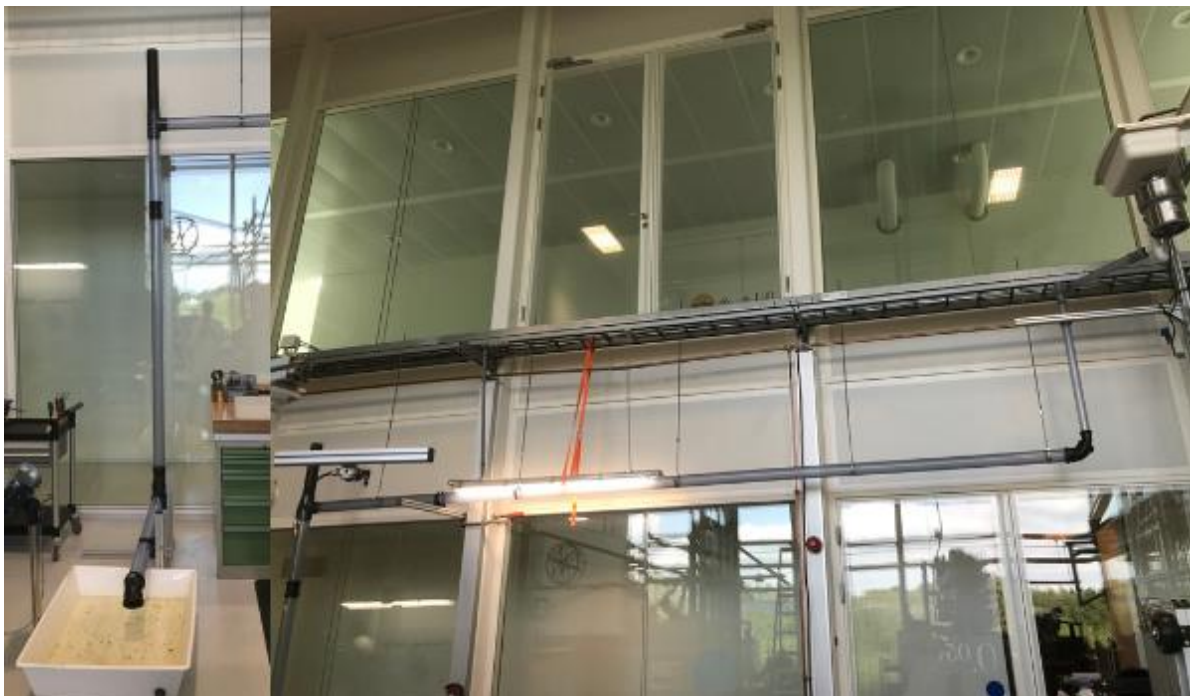
Figure 9 Indoor sewer configuration including 5 m horizontal collector pipe with 75 mm, vertical pipe (stack) of 2.4 m with diameter 75 mm, and horizontal bottom pipe of 1.3 m, 75 mm. Horizontal collector pipe Slope (1:50, 1:100, 1:200) and water flow rate (0.1 L/s, 0.3 L/s) varied according to the experiment carried out.
