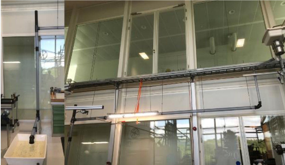
Figure 32 Indoor sewer configuration setup at KWR, including the vertical pipe.
